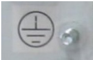
Fig. 27: Grounding stud marked with PE symbol
